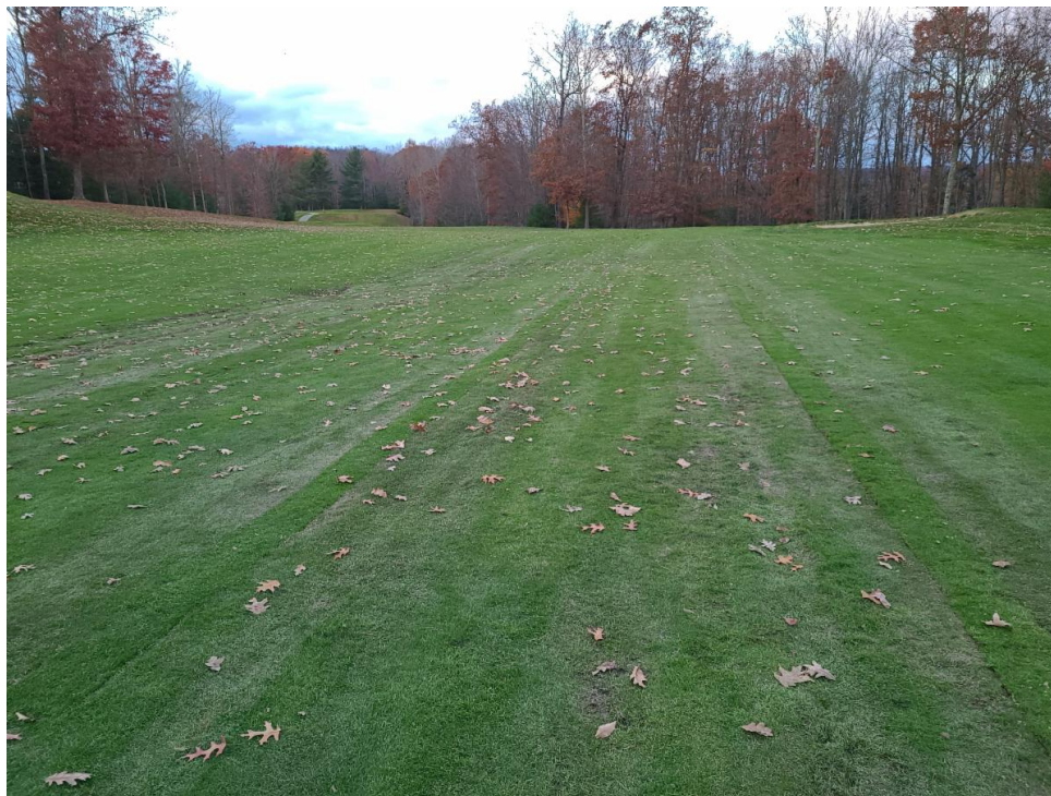
Number 7 fairway after drainage is installed and sod has been replaced.
