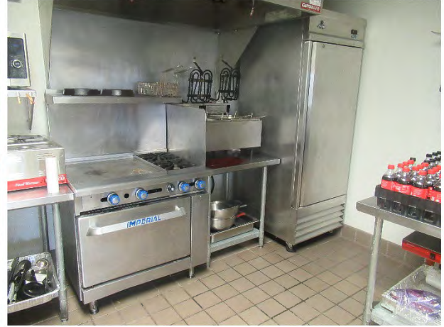
Kitchen equipment overview
