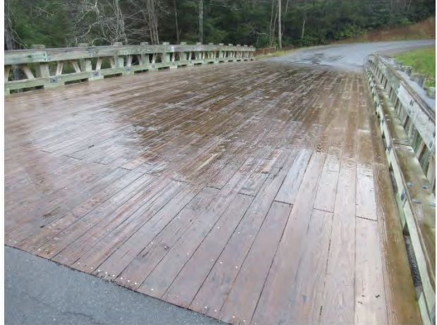
Glade Creek bridge decking
