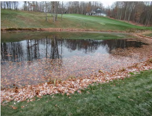
Pond at hole #4 overview – Note: Woodhaven Course
