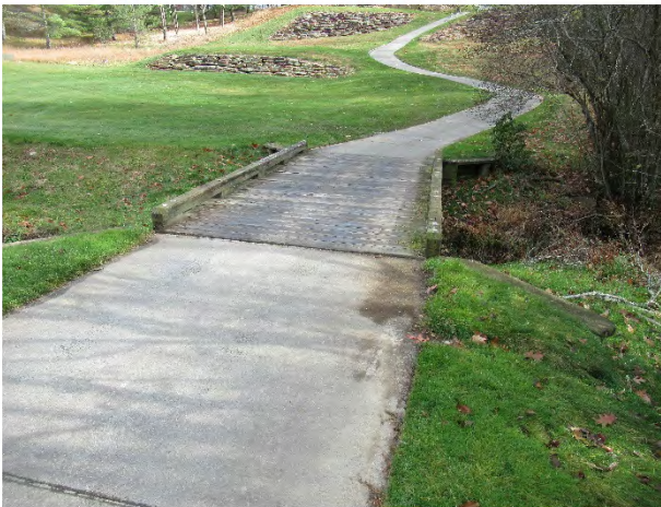
Wood cart path bridge overview – Note: Stonehaven Course
