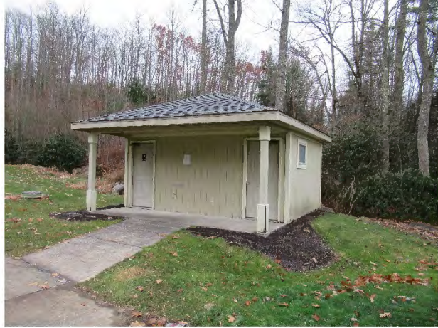
Rest room building overview – Note: Woodhaven Course
