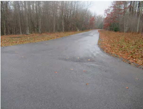
Asphalt pavement overview
