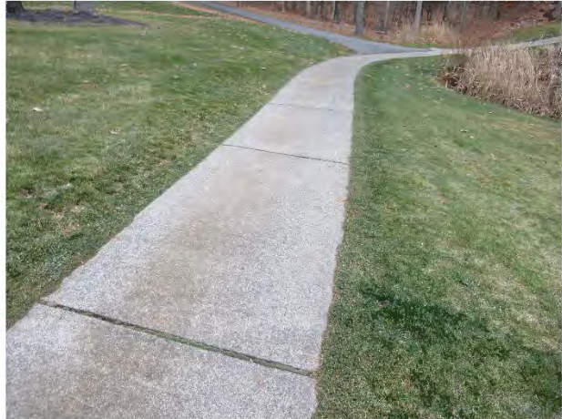
Concrete cart path overview – Note: Woodhaven Course
