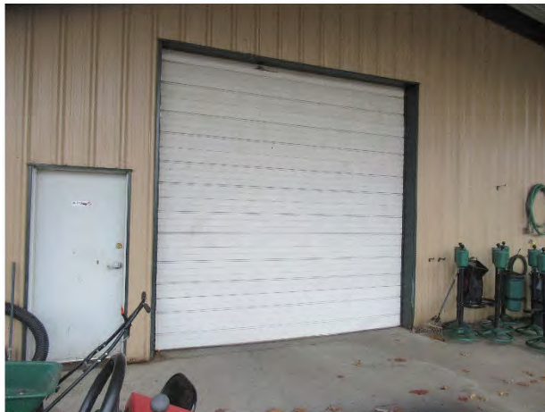
Overhead door – Note: Woodhaven maintenance building
