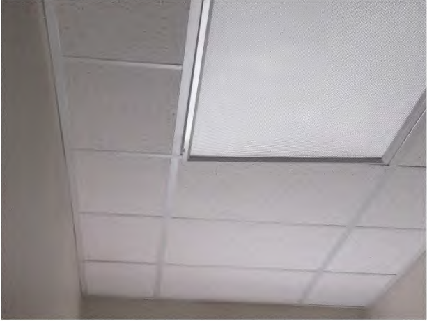
Acoustical ceiling tile and grid system – Note: light displacement
