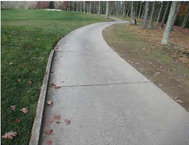
Concrete cart path overview – Note: Stonehaven Course
