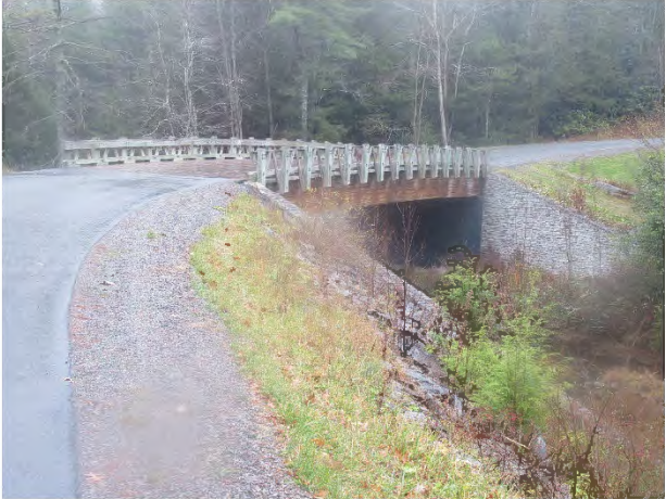
Glade Creek bridge overview
