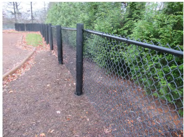
Chain link fence at playground
