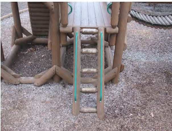
Playground equipment wear
