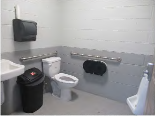
Starter building rest room overview
