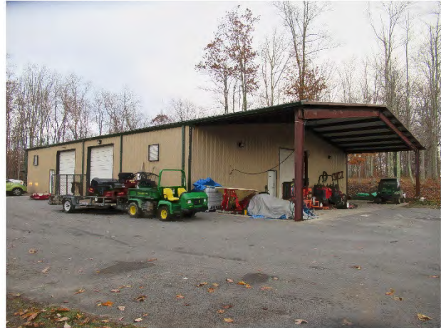
Woodhaven maintenance building overview
