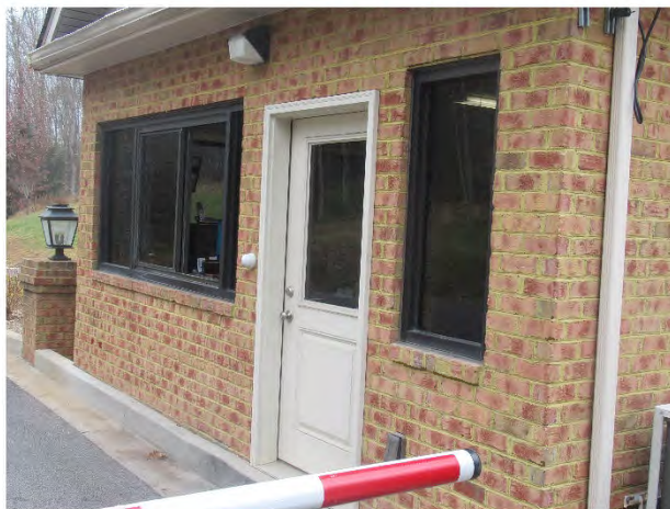
Windows and door at security gate house
