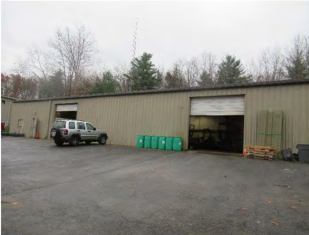
Stonehaven maintenance building overview
