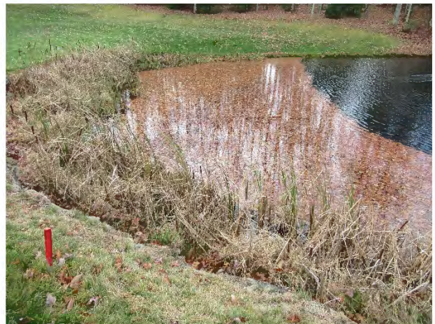
Sediment accumulation – Note: Stonehaven Course
