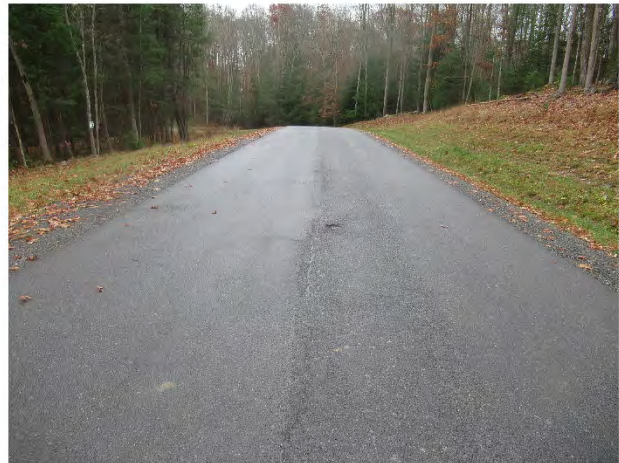
Asphalt pavement overview
