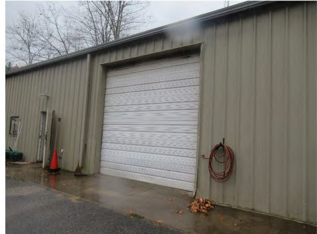
Overhead door – Note: Stonehaven maintenance building
