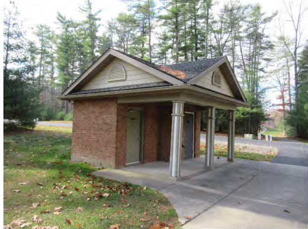
Rest room building overview – Note: Stonehaven Course
