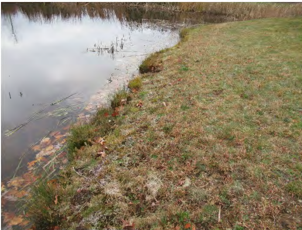
Minor shoreline erosion at hole #1 pond – Note: Woodhaven Course
