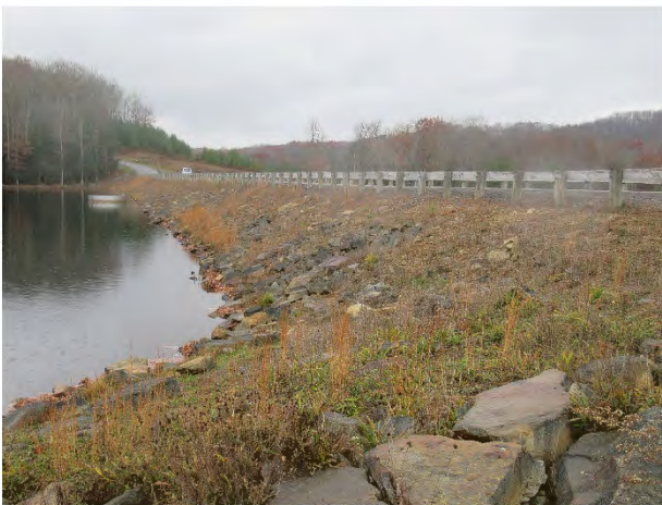
Earthen dam overview
