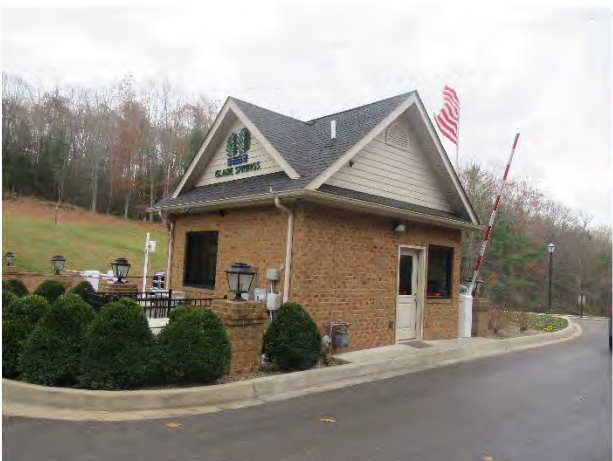
Security gate overview
