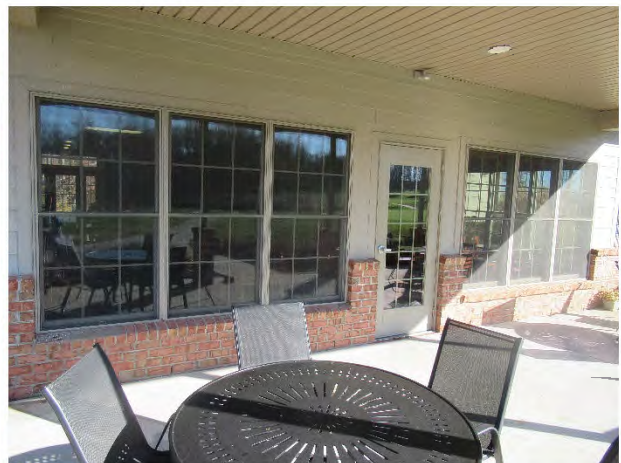
Windows and doors overview
