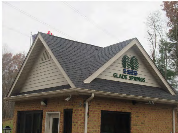
Asphalt shingle roof assembly at security gate house
