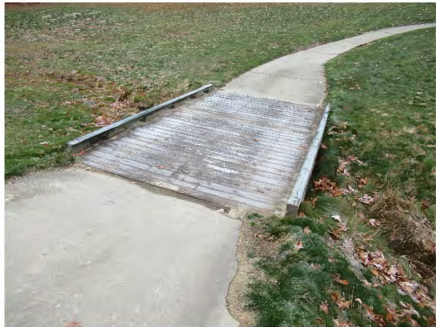
Wood cart path bridge overview – Note: Woodhaven Course
