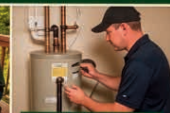
WATER HEATER INSPECTION
