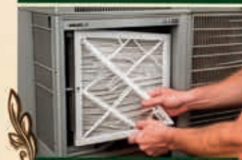
HVAC FILTER CHANGE
