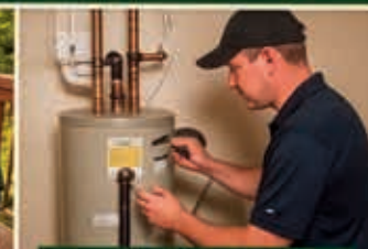
WATER HEATER INSPECTION
